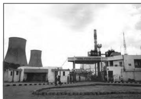
Fig 3.12: A view of a Thermal Power Station
