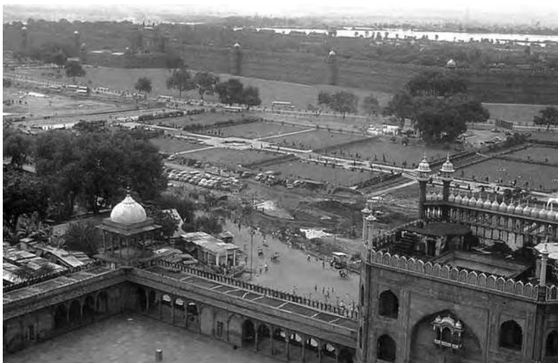
Fig. 8 – View from the Jama Masjid after the surrounding buildings were demolished
