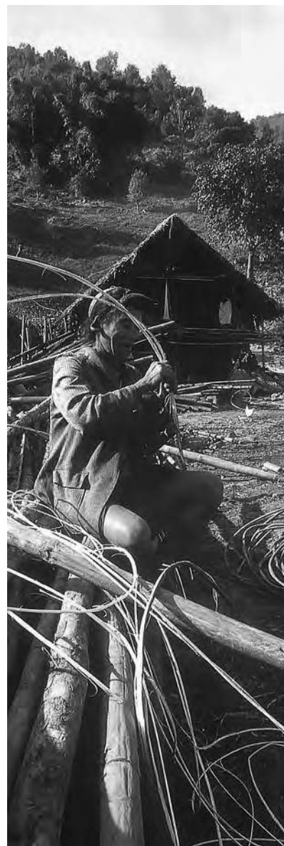
Fig. 5 – A log house being built in a village of the Nishi tribals of the Northeast.
