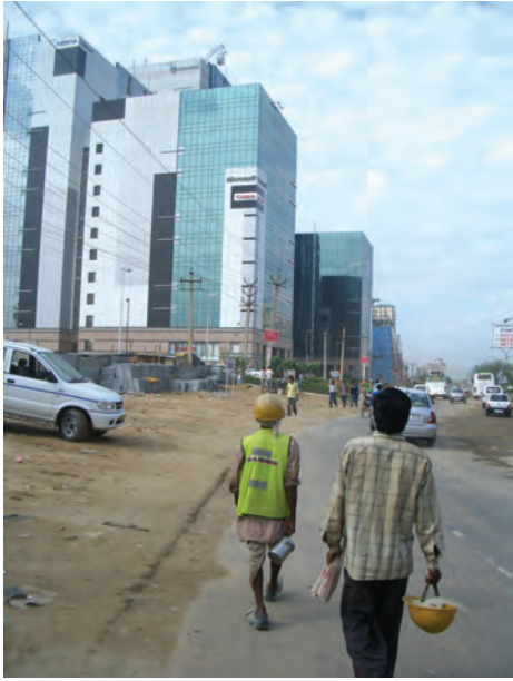
Accidents are common to construction sites. Yet, very often, safety equipment and other precautions are ignored.
