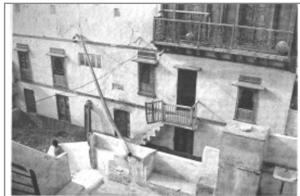
Rooftop harvesting was common across the towns and villages of the Thar. Rainwater that falls on the sloping roofs of houses is taken through a pipe into an underground tanka (circular holes in the ground), built in the main house or in the courtyard. The picture above shows water being form a neighbour's roof through a long pipe. Here the neighbour's rooftop has been used for collection of rainwater. The picture shows a hole through which rainwater flows down into an underground tanka .
