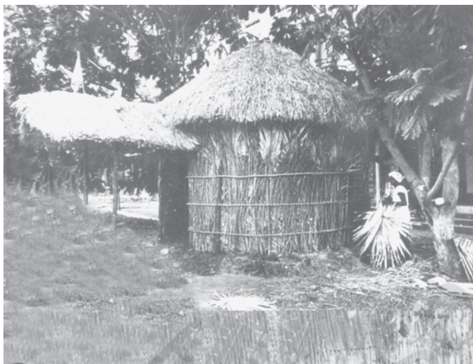
Fig. 4.2 Many poor families live in kutchas houses
